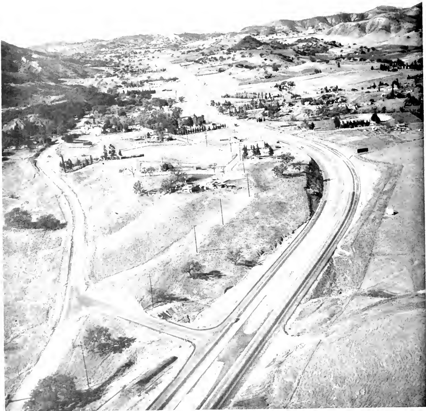
Looking westerly along completed section of Ventura Freeway through community of Agoura. Old state highway now used as local road on left.
